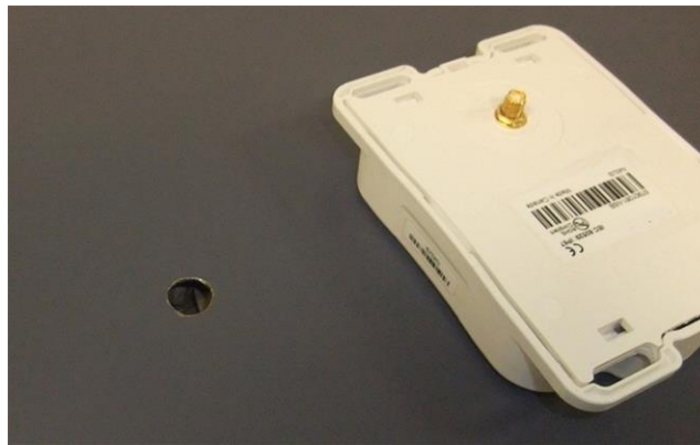
Figure 7: Drill Mounting Hole
